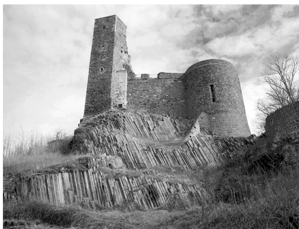
Fig. 1 – Stolpen Castle Hill – the type locality for the term “basalt” – with inclined basaltic columns at the western edge.
