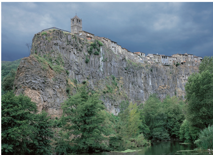
Figure 3. Photograph of the village of Castellfollit de la Roca. Credits © Turisme de la Garrotxa.
